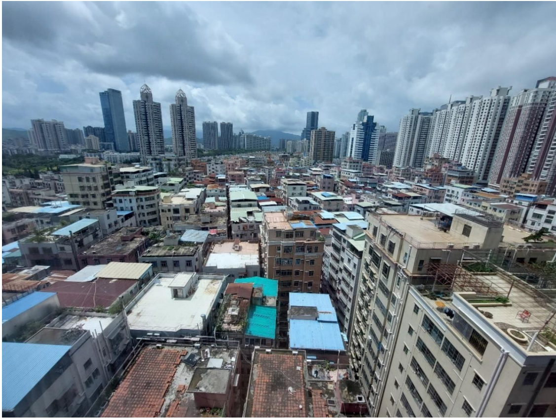
Figure 2. Bird view of Gangxia Village from North commercial side, showing the mid-rise residential towers in a densely-populated urban area (Source: The Authors).
