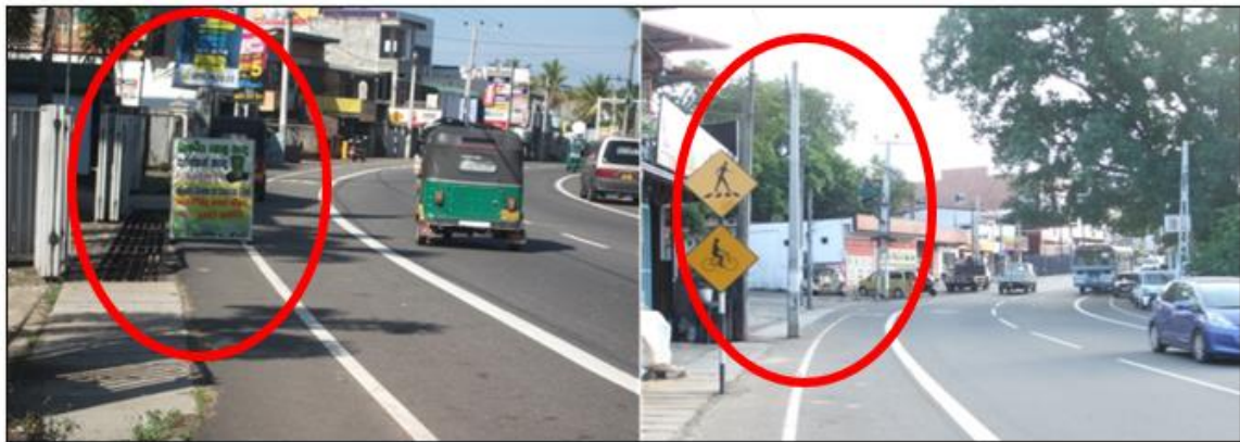
Figure 4: A sidewalk blocked by display boards and lamp posts Source: Public Domain
